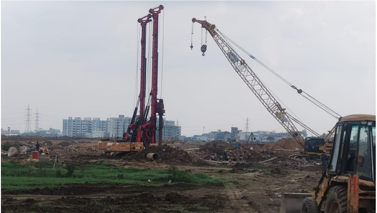
Fig.9: Piling in Progress in for Workshop area
