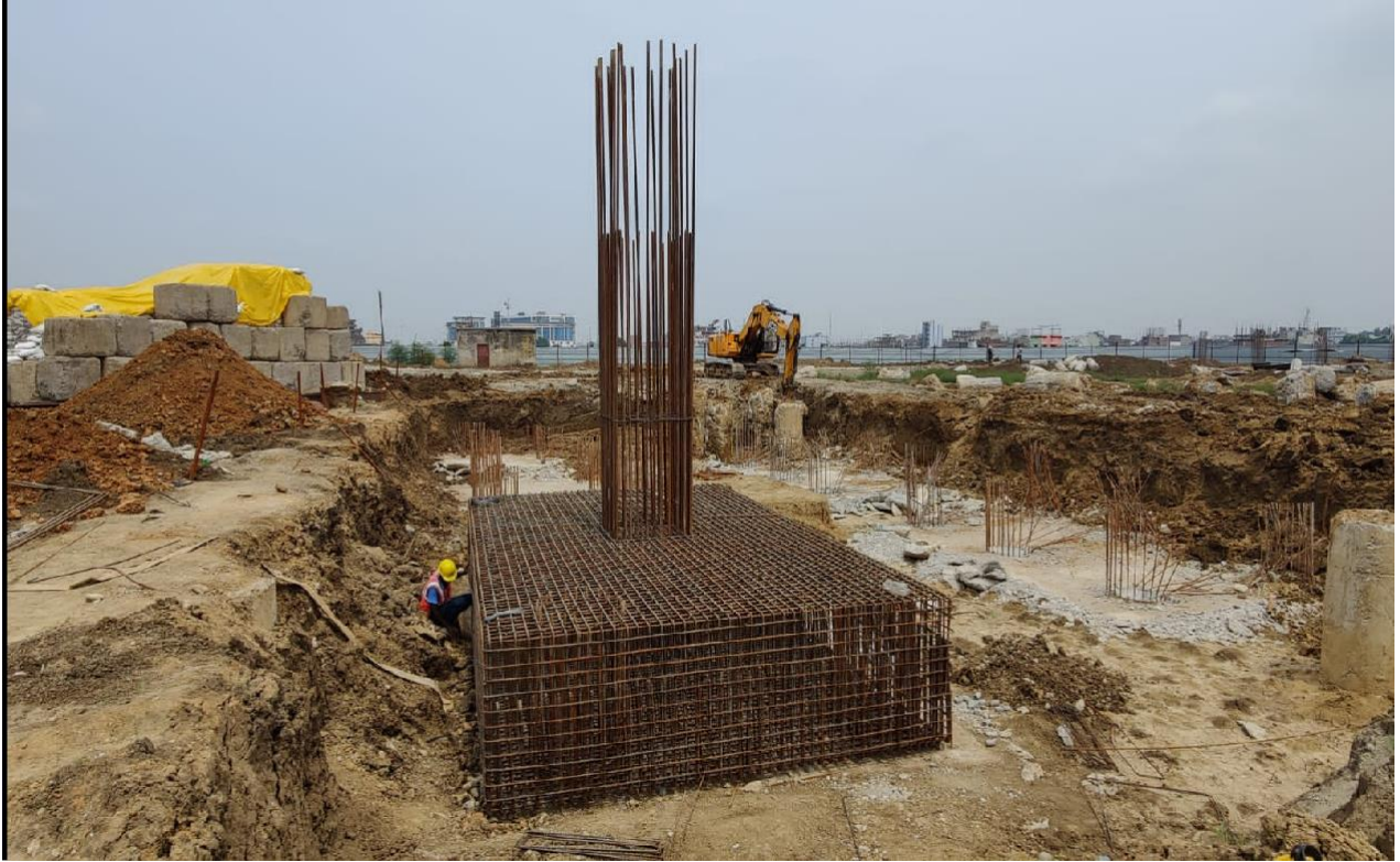
Fig.7: Admin Building Pile Cap Work in progress
