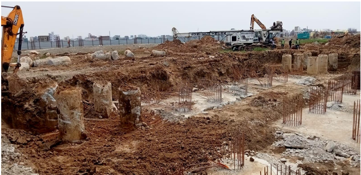
Fig.8: Excavation for Pile Cap in Progress in Admin Building area
