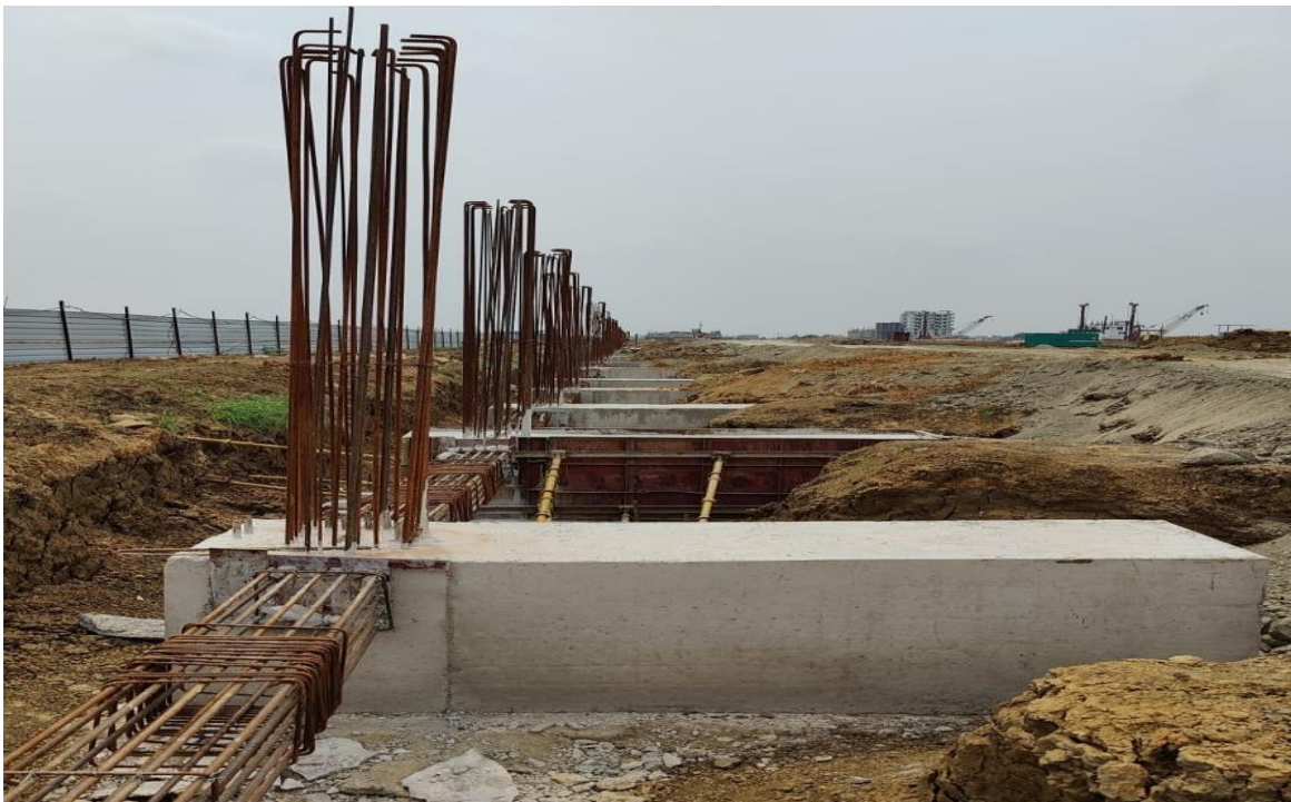
Fig.10: Boundary Wall Pile Cap Casting Opp. Badshahi Nala
